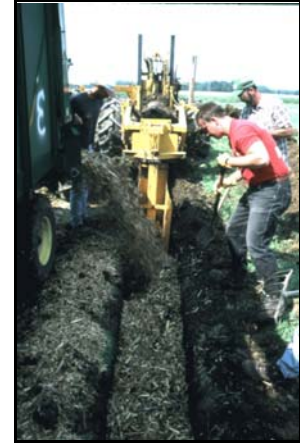
Fig. 6. Installing wood chip trench.
