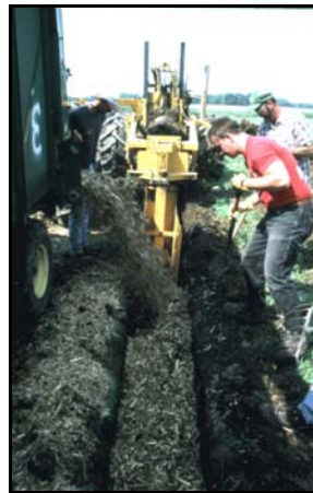
Installing wood chip trench.
